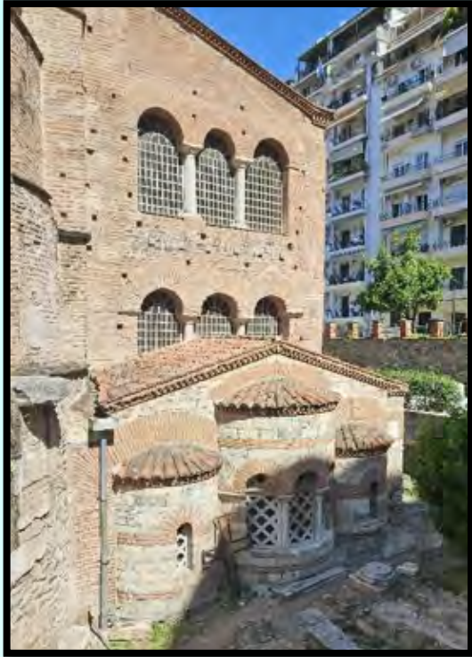
Photo 9 A New Church Built Over an Ancient Church, Thessaloniki, Greece
